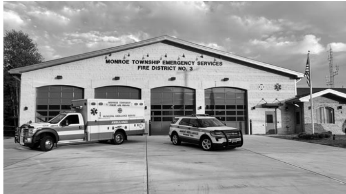
The new Monroe Township Fire District No. 3 firehouse located at 359 Schoolhouse Road will now be staffed 24/7 by Monroe Township EMS and equipped with the latest technologies to handle any emergency.
